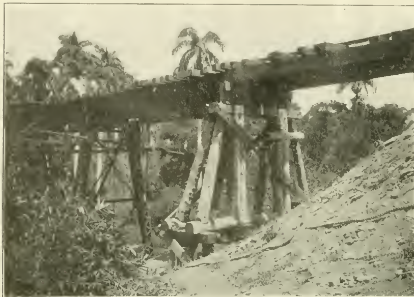
STEEL SPAN AND TRESTLE WORK, EASTERN DIVISION.
